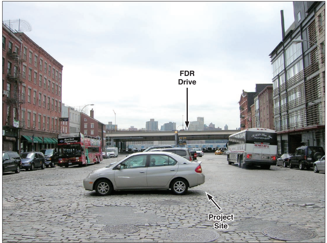
View southeast across project site 1
