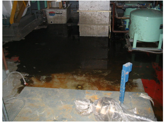
Figure 2 : Floor 40 water damage and mold.
