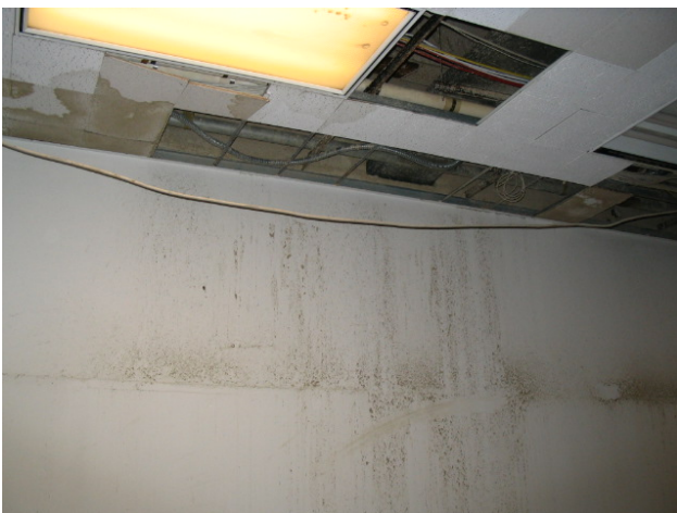
Figure 11: Floor 22 water damage
