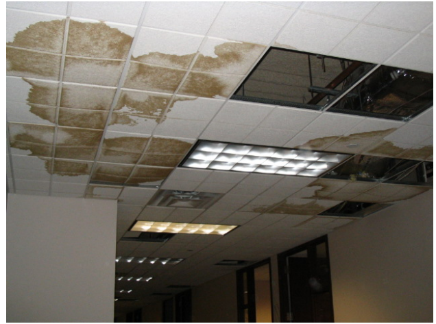
Figure 8: Floor 32 water damage
