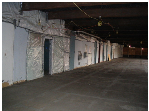
Figure 18: Floor 3 open area
