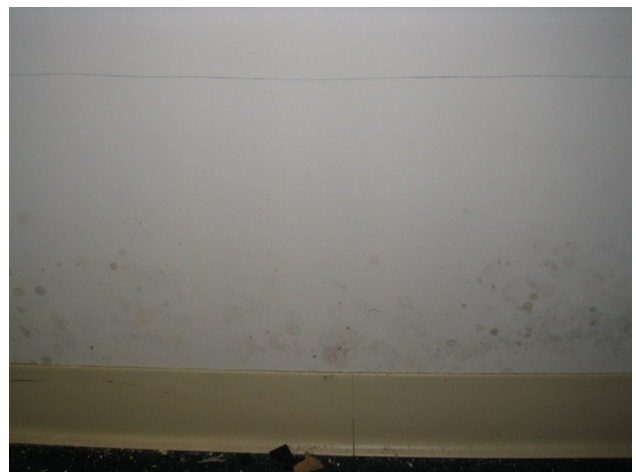
Figure 6: Floor 32 sheetrock mold
