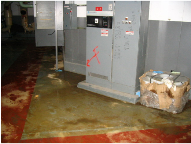
Figure 13: 5th Floor water damage
