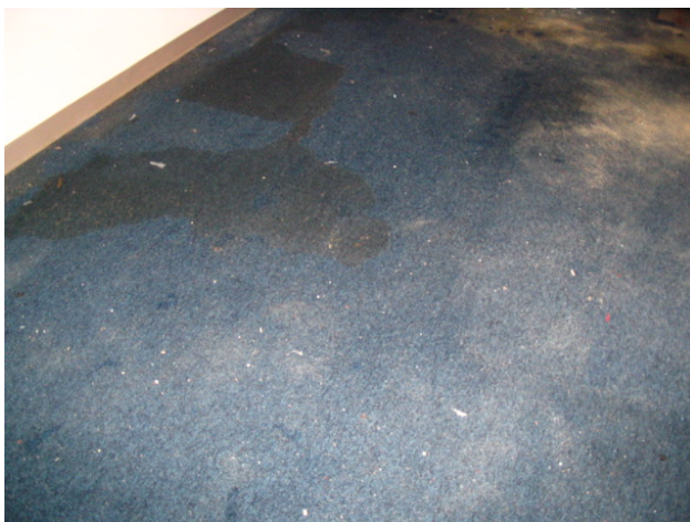
Figure 5: Floor 27 carpet water damage
