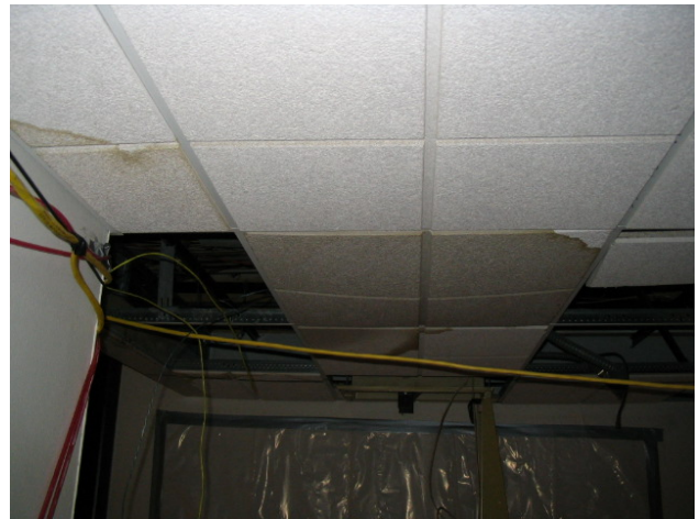
Figure 4: Floor 39 water damage.
