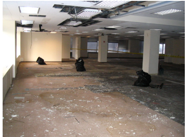
Figure 10: Floor 23 water damage
