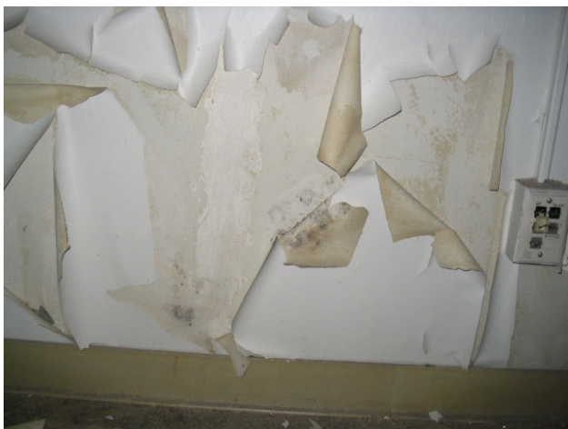
Figure 17: Floor 1 water damage
