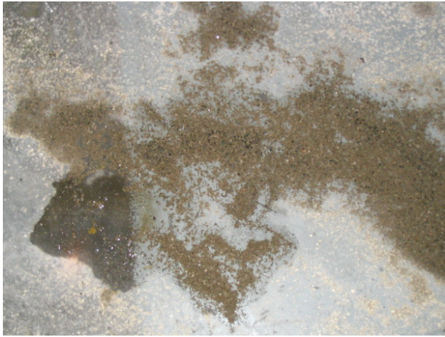
Figure 1: Floor 41 mold on flooring near pipe leak.
