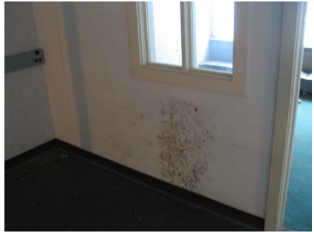
Figure 16: Floor 1 mold on sheetrock
