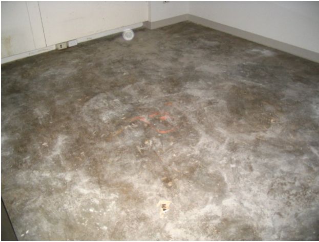
Figure 7: Floor 27 carpet water damage and visible mold
