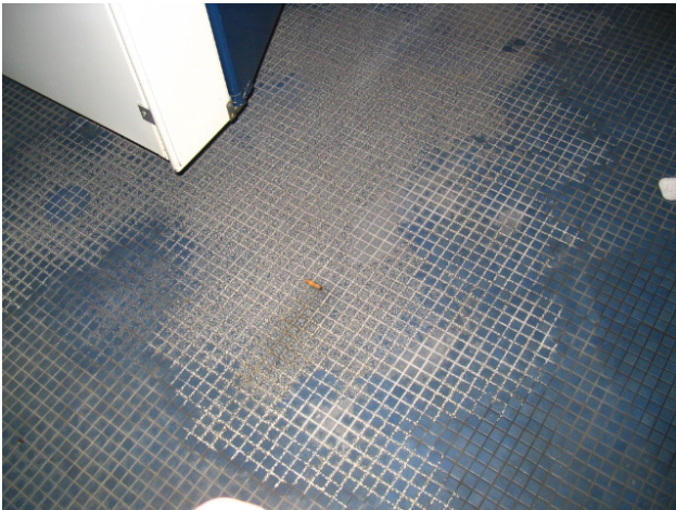
Figure 9: Floor 28 mold on flooring
