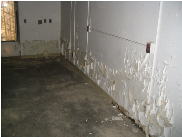
Figure 15: Floor 1 water damage
