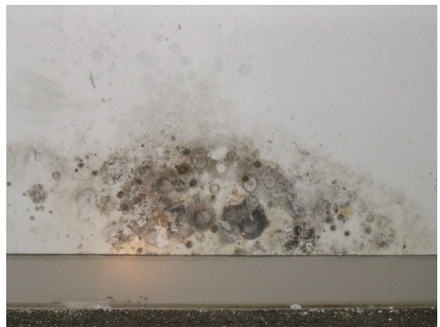
Figure 12: Floor 11 visible mold on sheetrock
