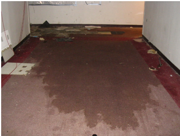
Figure 3: Floor 39 water damage
