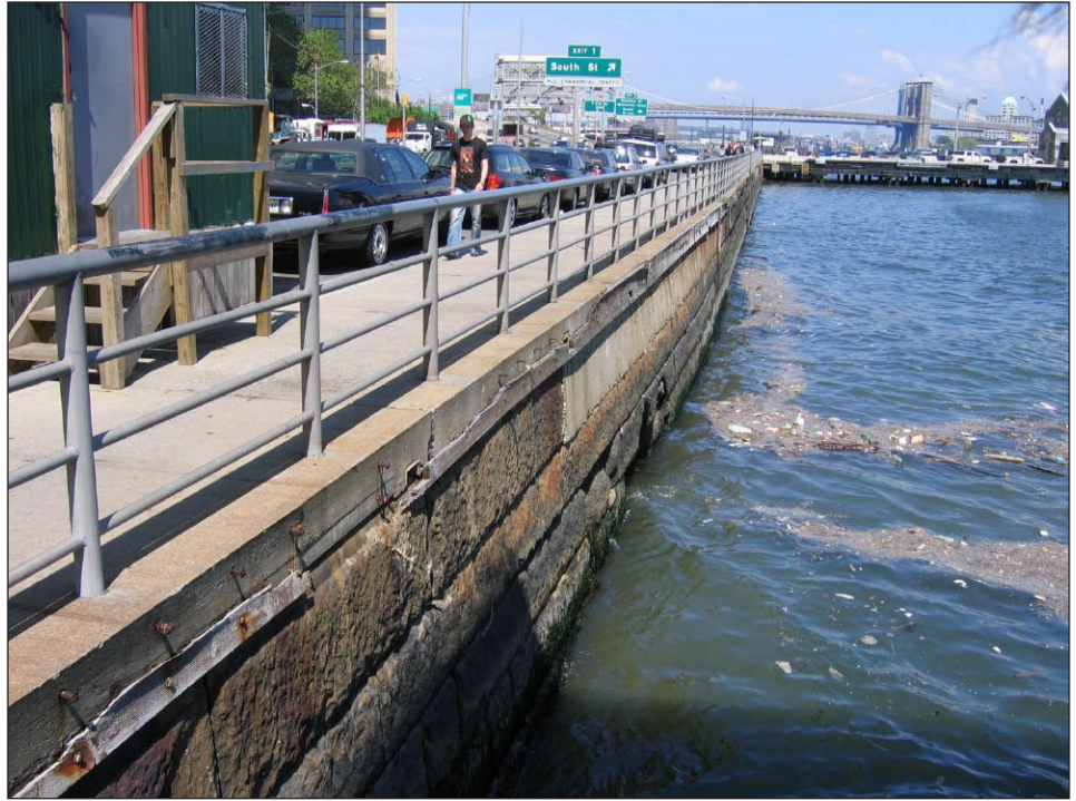
East River Bulkhead 6
