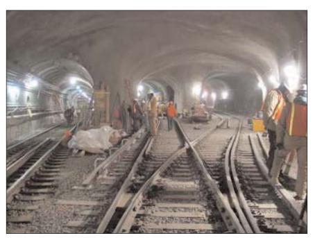
The Port Authority is creating new crossover tracks at Exchange Place in Jersey City to enable PATH service restoration at that station by June 2003.
